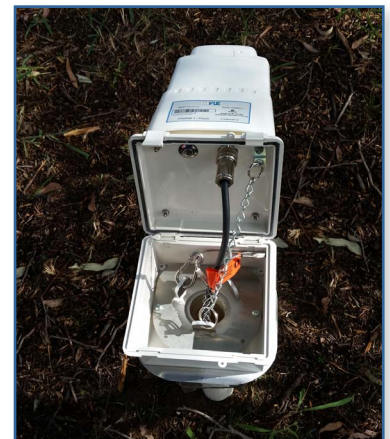
Submersible Level / Pressure sensor attached and lowered into the bore well.
